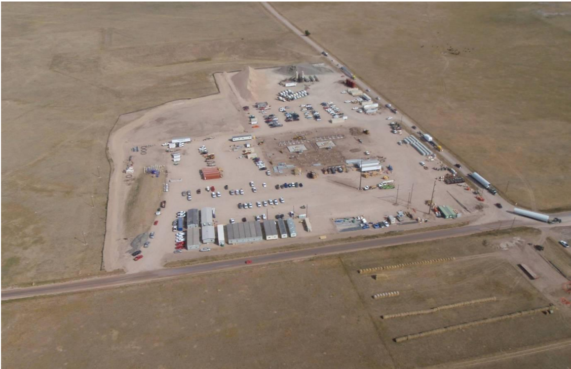
Figure 2-1: Typical Construction Laydown Area
