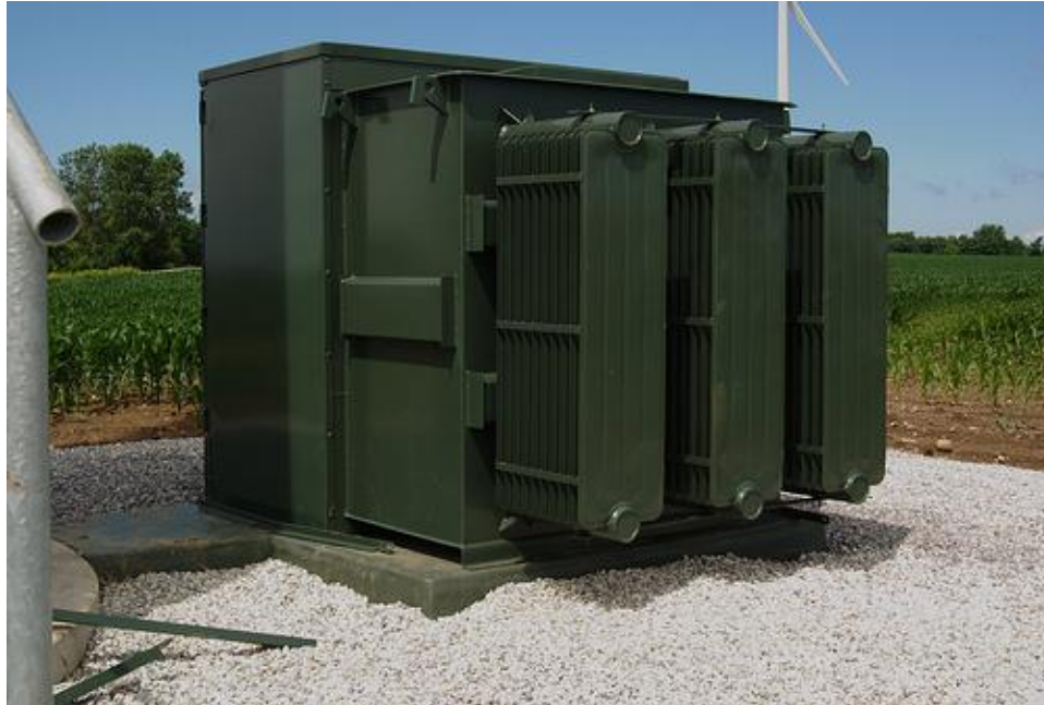
Figure 2-5: Typical Pad-Mounted Transformer
