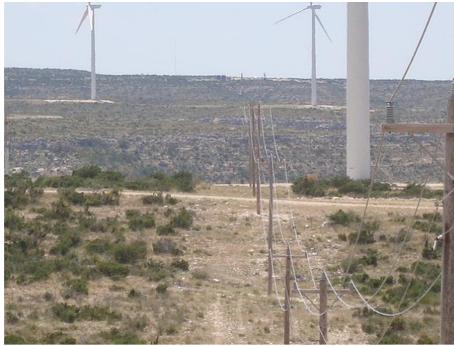
Figure 2-8: Typical Structures for Aboveground Collector Lines
