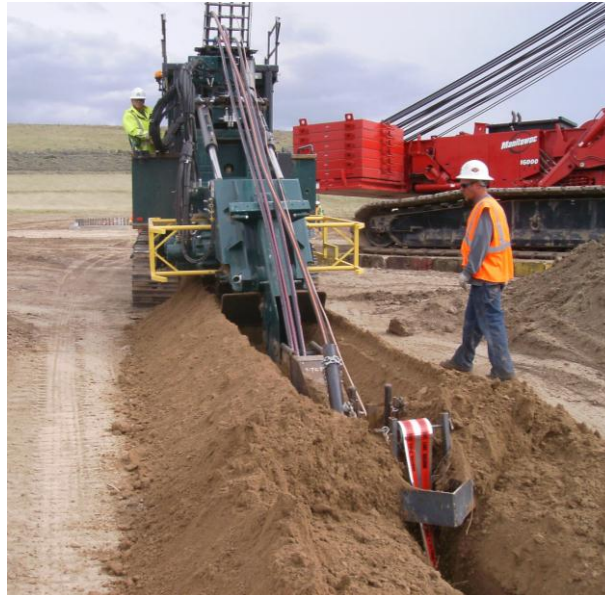
Figure 2-7: Typical Trench for Electrical Collection Cables
