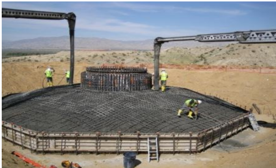
Figure 2-4: Typical Pouring of Turbine Foundation
